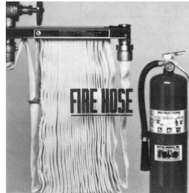
FIGURE A.3.3.19.4 Semiautomatic Hose Rack Assembly.
